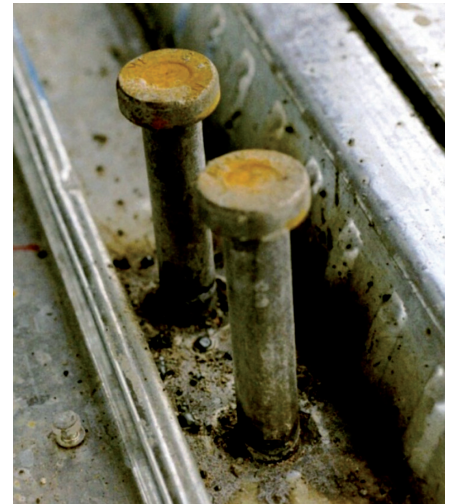
Figure 8: Headed studs welded through profile decks
