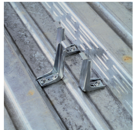
Figure 9: Hilti X-HVB installed in profile deck
