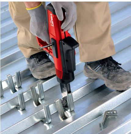
Figure 3: X-HVB shear connector with composite decking
